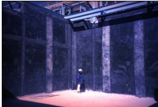
Figure 11. View of one component of the Tank Farm area.
