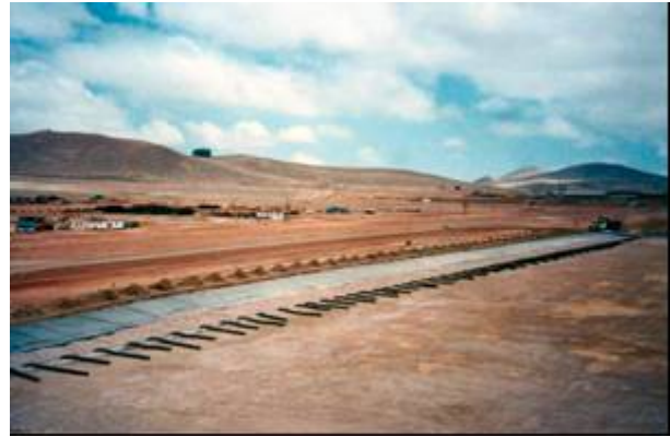
Figure 2. View of the collection system in a heap leach.
