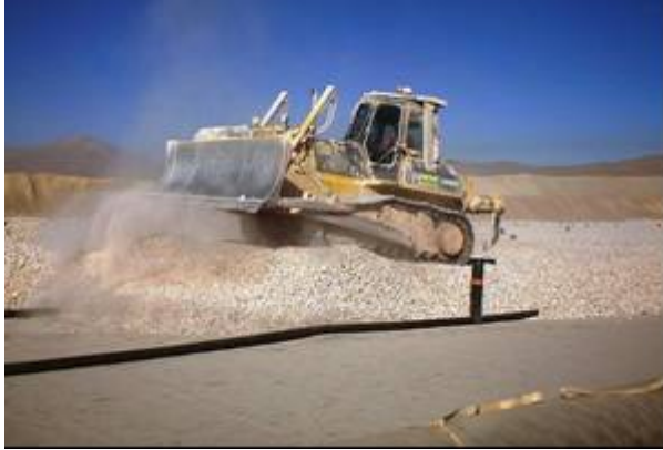
Figure 1. Protective layer installation in a heap leach.
