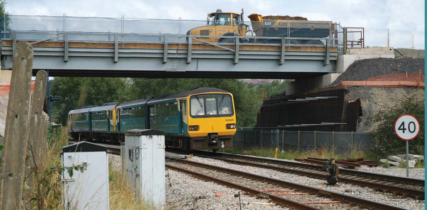
The Tensartech TR2 is often used to build low cost, temporary bridge abutments.
