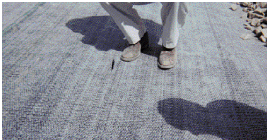
Photo 5: Top of GCL after loading.
