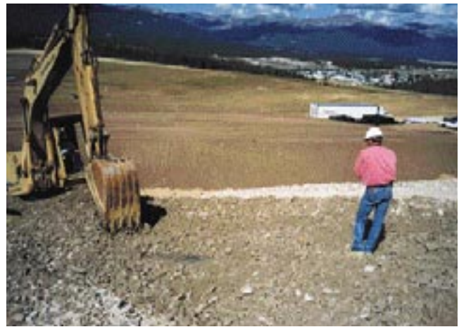
Photo 4: Removing rock cover
