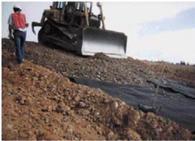
Photo 3: Spreading rock cover over geosynthetics
