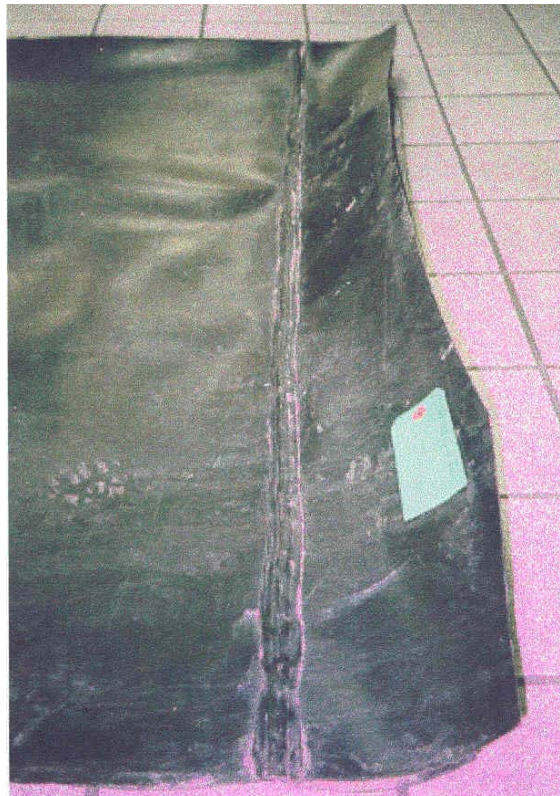
Figure 3: Welded Seam on Top Panel
