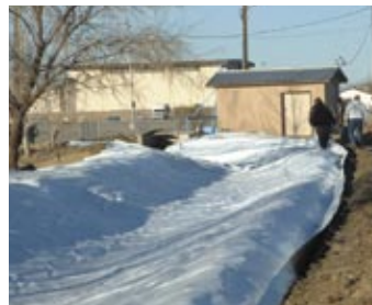
Exposed canal ditches
